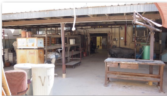
The West Deck before renovation...
